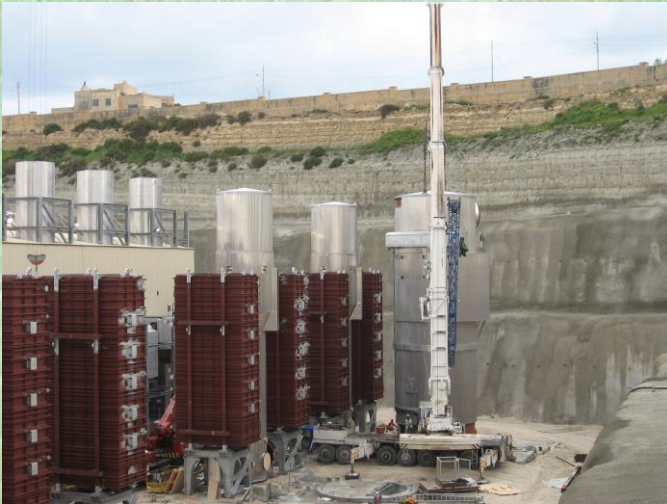
Installation of FILCON Bag Filter No. 1
