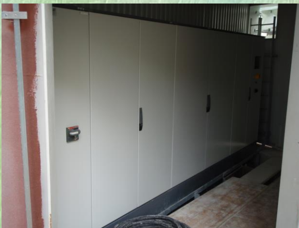
MCC and Control Cabinet – below the Filter module
