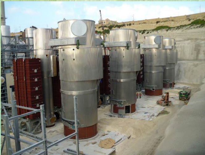
All 4 Filcon filters installed
