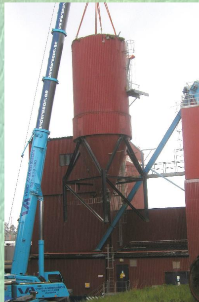
Spilt of the Reactor due to the weight (Build up inside)
