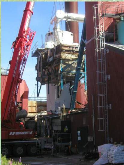
Dismantling of existent Bag Filter
