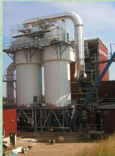
Installation of FILCON Bag filter No.2
