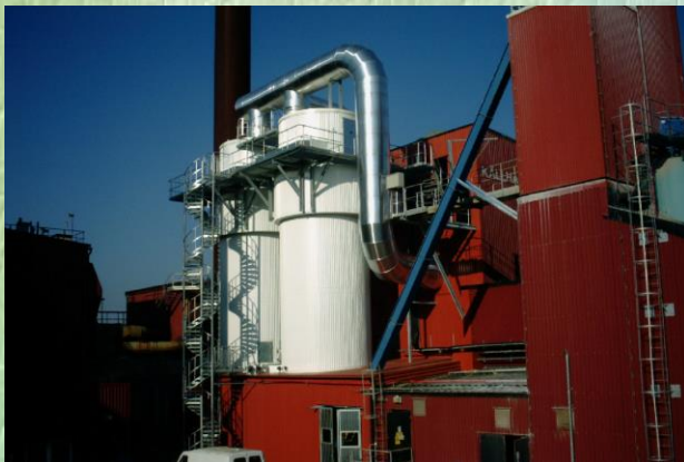
Final Plant, incl, Machine room for residue handling below the FILCON Bag Filters.
