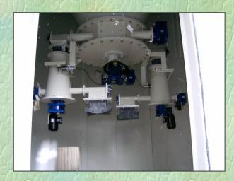
Hydrated Lime and Activated Carbon are injected into the flue gas duct before the filter for removal of acid components (SO2), heavy metals and dioxins.
